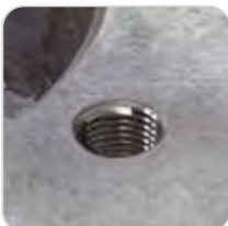
6. Thread is repaired and ready to use
